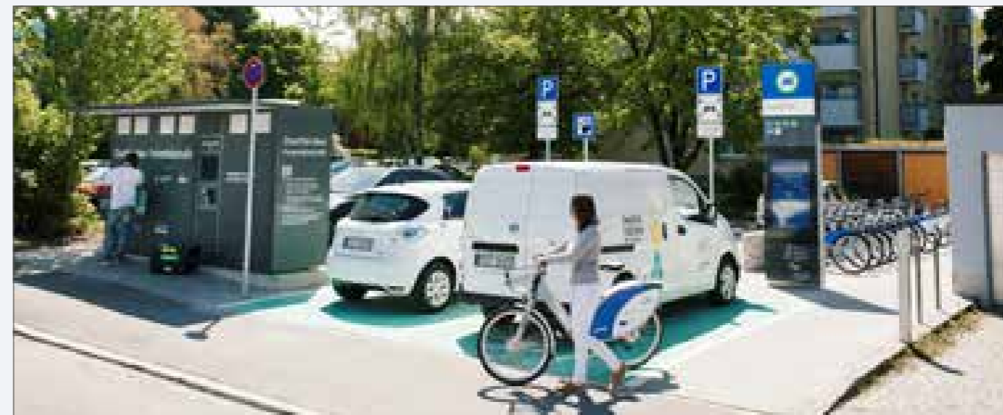
Mobility Hub Example showing electric vehicle charging, cycle hire, information board, drop off/collection facilities - Munich
